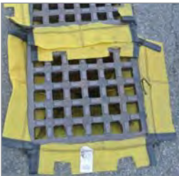
Silt bag drop inlet protection Image BSC Group
