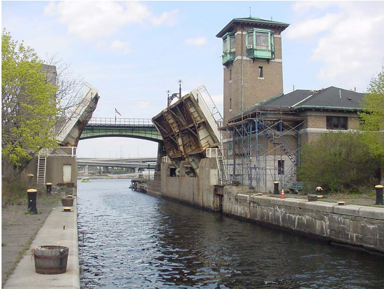
Craigie Drawbridge Rehabilitation Project
