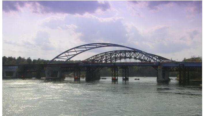
*View of completed steel arch on the new northbound span with existing Whittier Bridge in the background (May 2015)*
