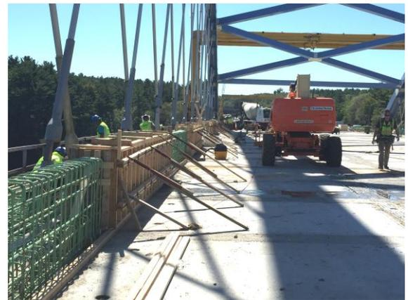
*Crews install structural steel and formwork for barriers on the Whittier Bridge in September 2015*
