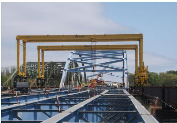
*Crews use a traveling gantry crane (yellow) to erect steel girders on the southern end of the new Whittier Bridge northbound span*
