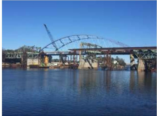
*Demolition of the old Whittier Bridge began in January 2016 and will continue through the spring. Once demolished, the new southbound span will be constructed in its place.*
