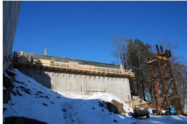
*Completed northern abutment for new Whittier Bridge northbound span*
