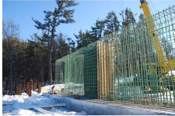
*Construction of southern abutment for new Whittier Bridge northbound span*
